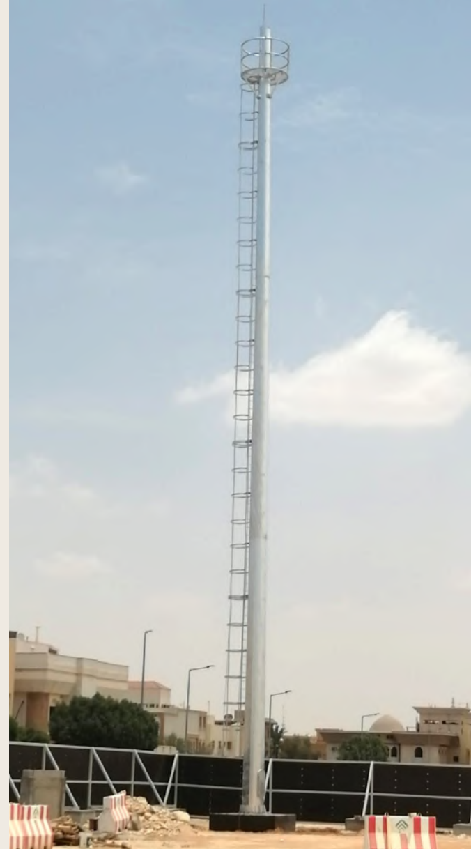
30M SECURITY TOWER WITH LADDER & PLATFORM SUPPORT
