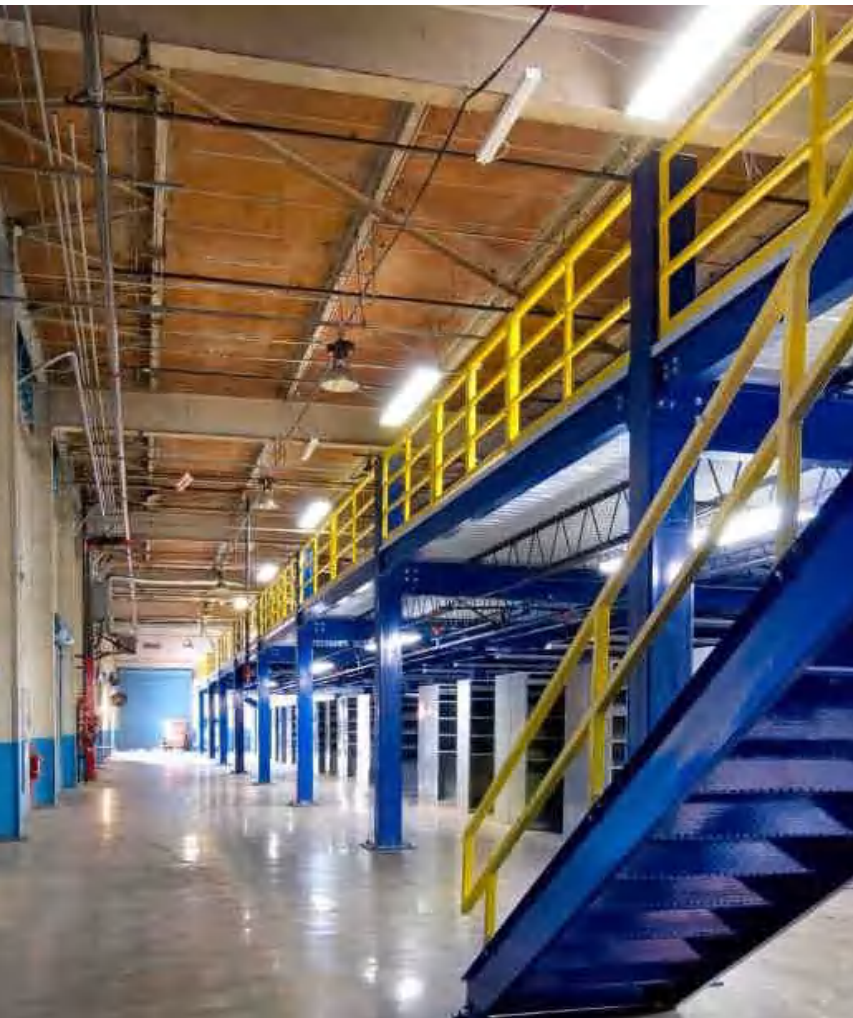
Hand Rails with steel Platforms
